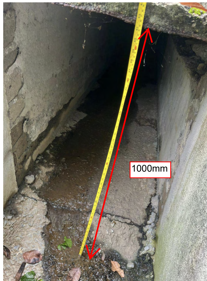
Dimension of 1000mm Box Culvert
