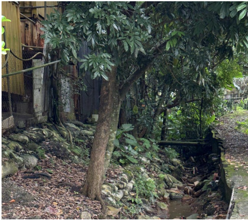
SITE PHOTO 8 EXISTING 3m x 2m existing channel
