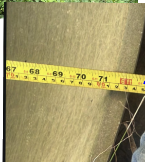
SITE PHOTO 7 EXISTING UNDERGROUND 830mm dia. PIPE and Existing Stream
