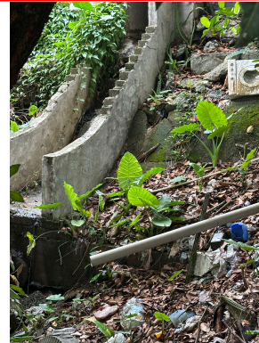
Fig Photo 1b: Stepped Channel and Existing Stream (3m (W) x2m(H))
